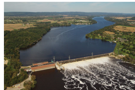
Prairie du Sac Hydroelectric Project
