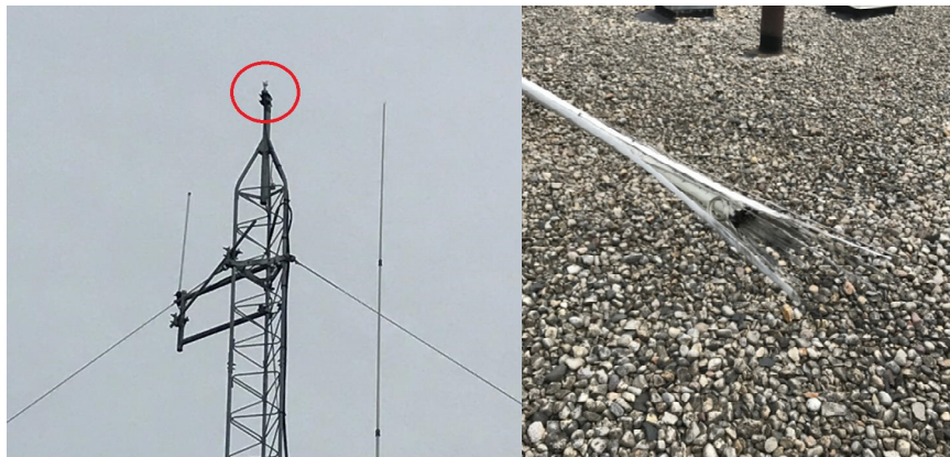
Figure 4.10.3: Two-Way Radio Antenna, hit by lightning, blown off the tower.
